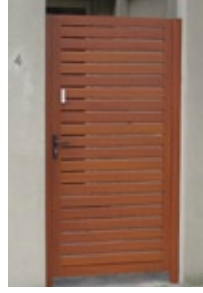
Horizontal timber finish on privacy screen and gate.
